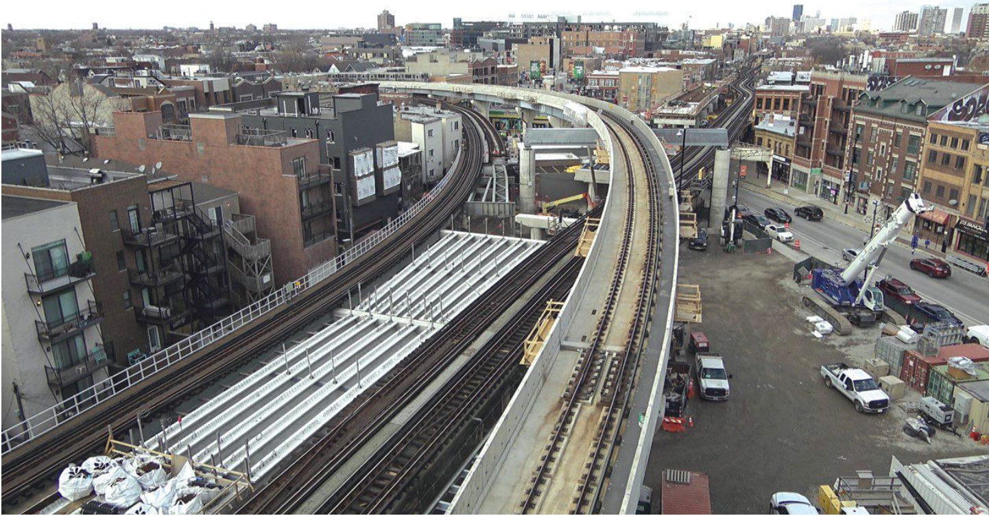
The north mainline construction for tracks 1 and 2 under the flyover structure. This view shows, from left, the temporary tracks; the precast, prestressed concrete beams that will carry tracks 1 and 2; tracks 3 and 4 on the existing structure; and the tracks on the flyover structure. Photo: Chicago Transit Authority.
