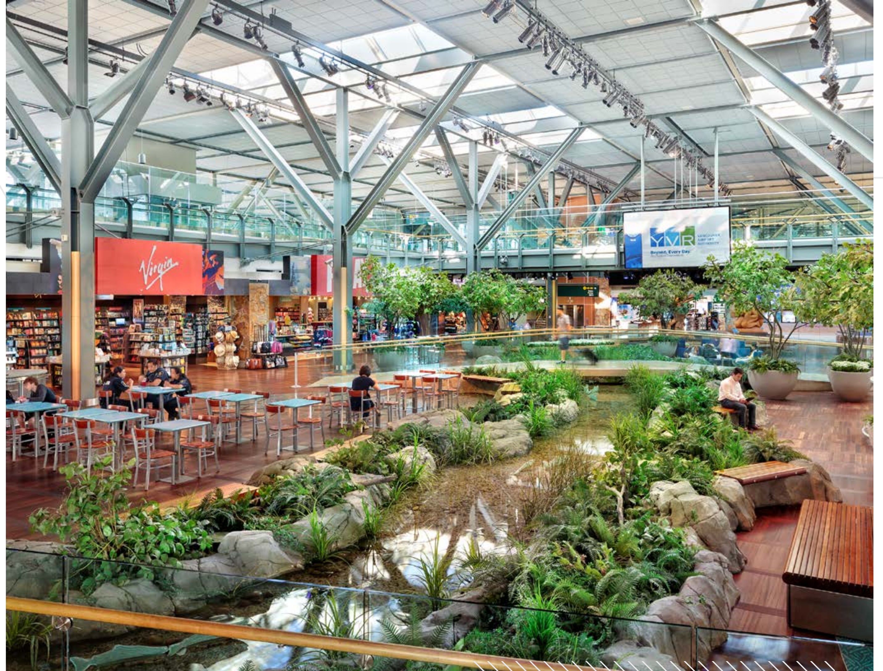
📍 Vancouver International Airport - International Terminal West Chevron Expansion Richmond, BC
